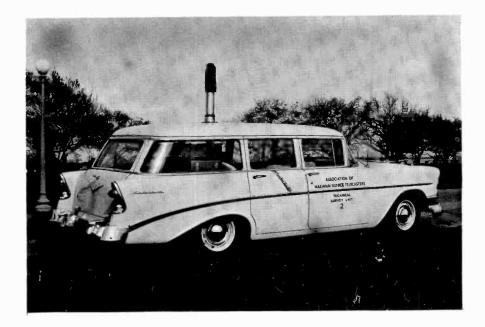
Figure 1 - MST Mobile Survey Unit No. 2. The hydraulic mast is shown in the retracted position for traveling.
