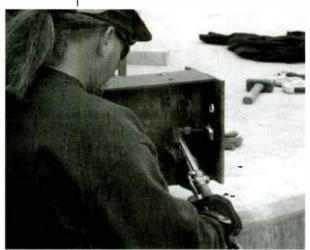
A worker enlarges anchor holes on the transmitter building support beams.<sup>1</sup>
