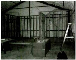
Insulation has been blown in and the framing is in for the bathroom and studio areas.
