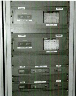
The HD rack sits between the transmitters. Each transmitter has its own HD exciter.
