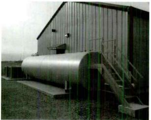
The 4,000 gallon diesel tank in place.
