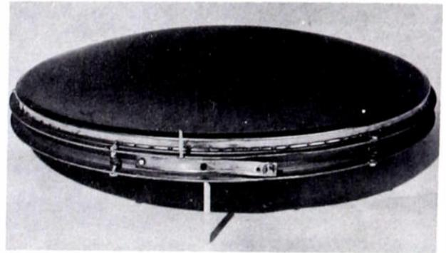
Fig. 4. Storage target assembly.
