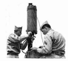
Amplifiers like this are used every 534 miles in the cable portions of the system. They are weatherproof, can be used on a pole or the ground; and will ever work under water. The system uses a spiral wound cable developed by the Signal Corps.
