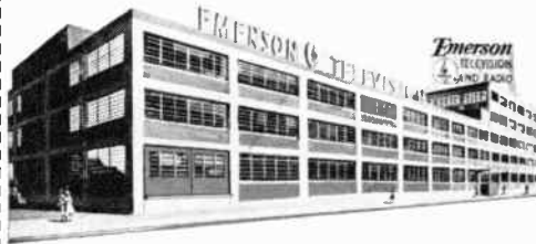
Emerson's new air-conditioned Main Office and Engineering Laboratories, Jersey City, New Jersey.
