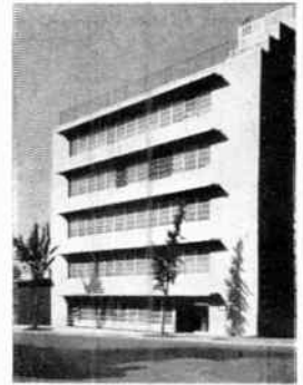
Emerson's new air-conditioned Research Laboratories Washington, D.C.
