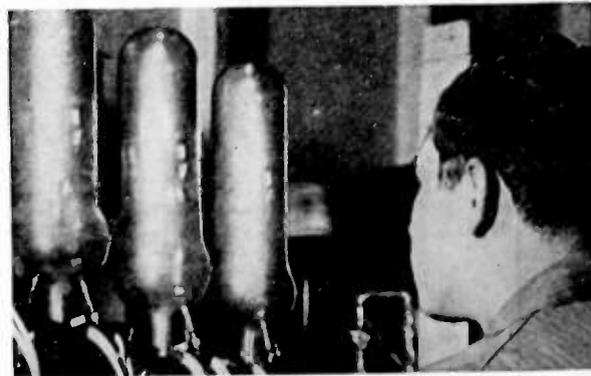
**FLASH FILAMENT TESTER** checks filaments before tubes are assembled and pumped. Here tubes are placed under a temporary vacuum, heated to much higher temperatures than will ever be required in normal use. Only perfect filaments reach the final stages of manufacture.
