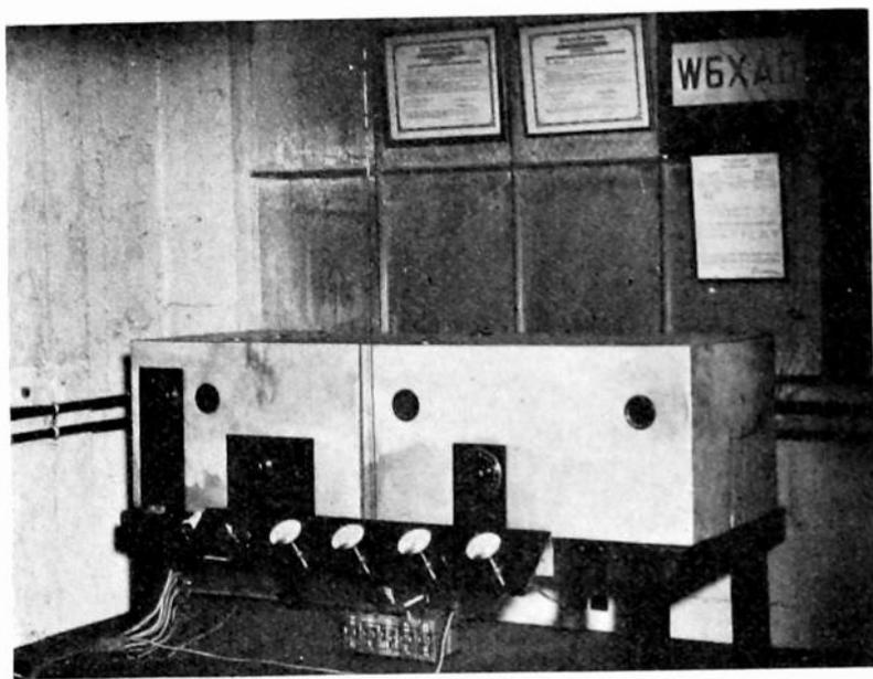
Fig. 1—Don Lee Broadcasting System television transmitter W6XAO—44,500 kc. Don Lee Building, Los Angeles, California.
