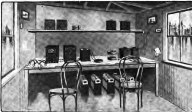
Interior of Static Eliminator Station
