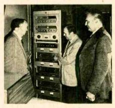
This shot of the audio control room at Notre Dame Stadium shows the four Crown DC-300A amplifiers, as well as the Spotmaster 5 BEM-2005 audio console and Crown VFX-2 filter.
