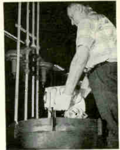
TUBE ASSEMBLY is removed from furnace making metal-ceramic seals
