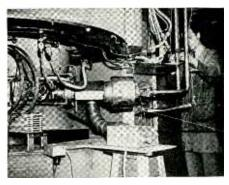
A scientist in the Royal Society Mond Laboratory of Cambridge University is making adjustments on a cyclotron machine. Neutrons, produced by the cyclotron, may be used as a substitute for radium
