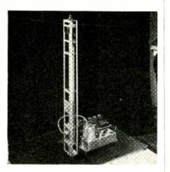
Reverberation device which uses a spring for sound transmission
