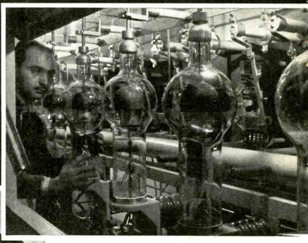
High-voltage rectifier arrangement which obviates manual changing of tubes during broadcast periods. In the background are relays for electrical changing of tubes.
