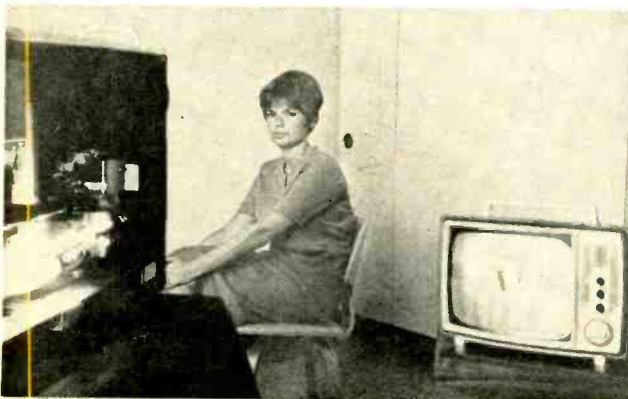
Light on or off, an image of the model appears on the television monitor. Illumination comes from a rapidly scanning laser beam that's virtually invisible to a person in front of the camera.
