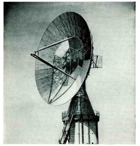
Typical scatter terminal equipment employing high-power klystron for ssb operation
