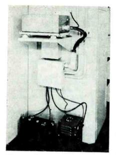
Typical installation of 60-watt f-m transceiver equipment in caboose
