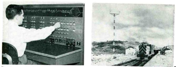
Dispatcher at console in Puerto Ordaz (left) controls switch positions at remote sidings by radio. Both track switches and signal lights are radio activated and each siding has a radio telephone for maintenance personnel
