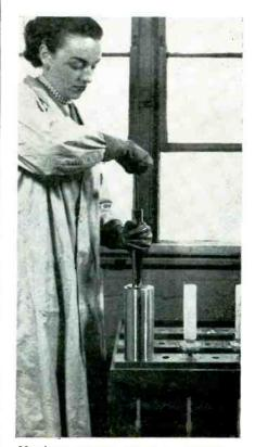
Metal can provides support for applicator while pushing down on plunger to force foam into antenna cavity. Scotch tape holds paper in position on antennas awaiting filling, to prevent surplus foam from overflowing down outside
