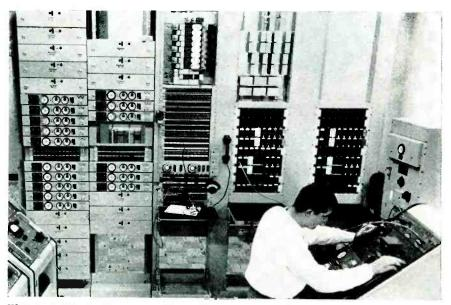
Western terminal equipment at Clarenville, Newfoundland of submarine cable that links North America with British Isles. Increased use of radiotelephone circuits and occasional radio blackouts made use of cable necessary. Fifty-one vacuum-tube repeaters built into the cable amplify signals every 40 miles. The facility is operated by Eastern Telephone and Telegraph Co., a Canadian subsidiary of A. T. & T.
