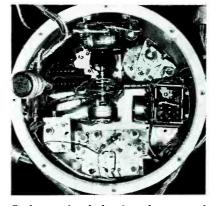
Rocket warhead showing placement of units. Beacon is circular can at upper right. Function selector switch at center is for prefiring check
