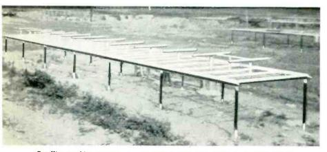
Satellite tracking antenna is mounted on jack-type posts to permit leveling
