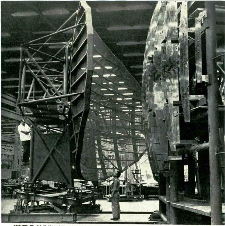
PRECISION JIG (RIGHT) GAGES ACCURACY OF HUGE ANTENNA SURFACE TO 1/100 OF AN INCH-PROOF THAT LARGE OR SMALL ....
