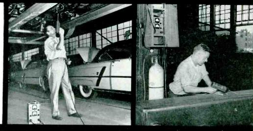
**IN ASSEMBLY-LINE TESTING** of Lincoln automobile air-conditioners, the General Electric Halogen Leak Detector, Type H-1, is used to quickly "sniff" all vital connections under the chassis and hood. TO CUT REJECTS, the Angle Products Company, Cleveland, Ohio, checks their hydraulic oil and fuel tanks with the G-E leak detector. It has reduced the company's inspection time by 35%.
