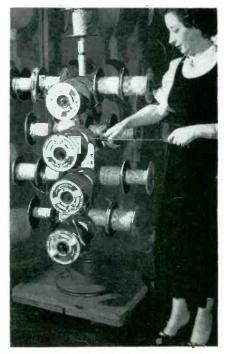
Removing length of wire from spool on tree. Dolly permits moving entire tree readily to input end of Artos machine when desired
