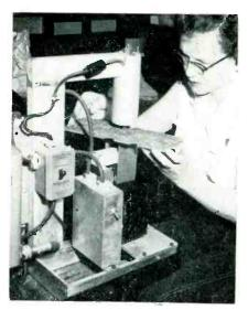
Hot staking setup for anchoring eyelets in holes of printed wiring board
