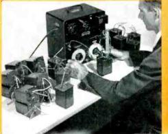
Checking Center-Tapped Windings Impecances on either side of a center-tapped winding are accurately compared to insure the tap is correctly centered. The winding ends are connected to the "unknown" and "stancard" terminals; the center tap goes to either ground terminal. The bridge then directly indicates the extent to which the turns on one side exceed those on the other.
