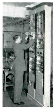
Relay station equipment undergoing tests prior to installation in the Alps
