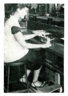
Foot-operated installation of lead-tailoring machine on assembly bench in typical electronic assembly plant
