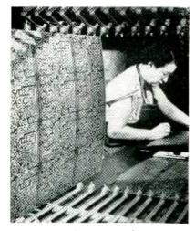
Inspecting etched wiring boards, produced twelve per sheet, and retouching where needed. Sheets are later cut, trimmed and punched. Molded plastic supports hold the sheets at top and bottom while drying
