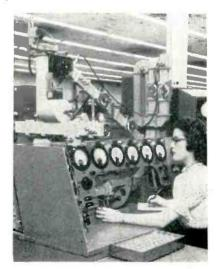
Production test set for microwave tubes
