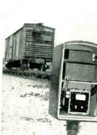
OPERATOR in freight-yard control tower (left) engages remote car-retarder when speed meter (right) warns that coupling speed is unsafe as . . .
