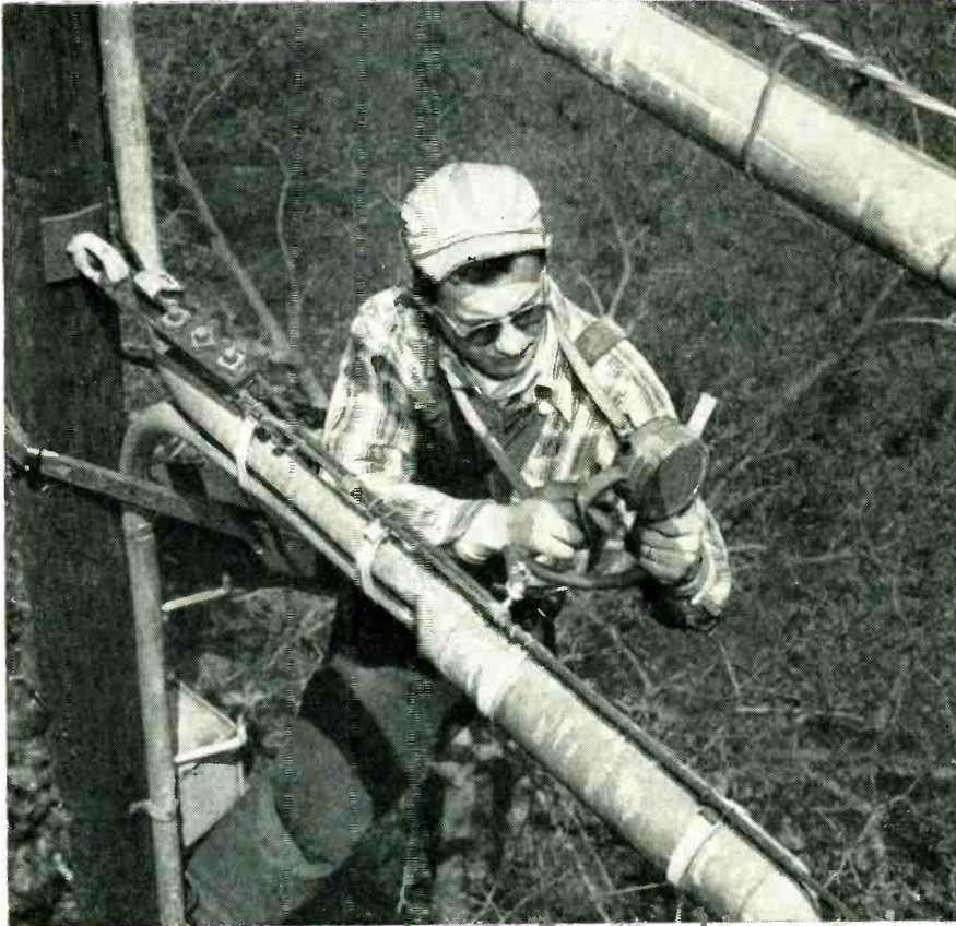
Air compressor and tank are at right. Long cylinders on rack dry air before it enters cables.
