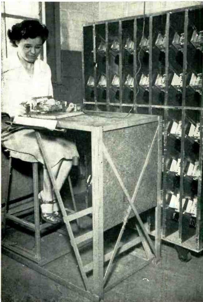
Tuner-storing rack and movable inspection table
