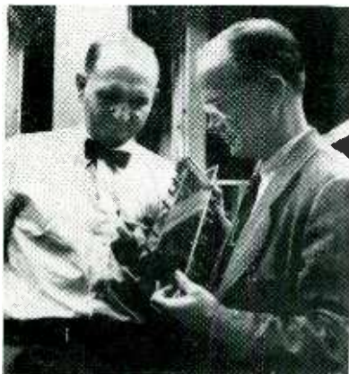
Long-distance dialing service in Englewood, N. J., is a Bell Telephone proving ground for transistor oscillator equipment. The oscillators are used to generate electrical signals by called numbers sent from one central office to another. Each oscillator unit uses six transistors
