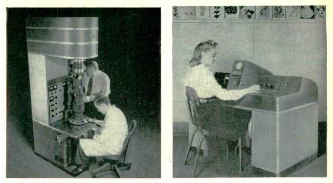
Early commercial model electron microscope type EMB, and the console type EMC that came along a little later
