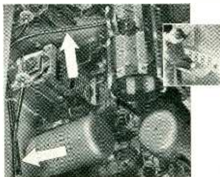
CENTRALIZING CONTROLS for more convenient operation is a simple matter when S.S. White shafts are used to link variable elements to their tuning knobs. This broadcast transmitter provides an excellent example.
