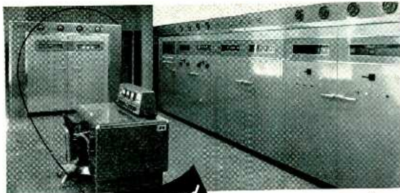
KFRE, Fresno, California. Front view of 50 kw AM transmitter control console and Johnson cabinet containing phasing equipment.
