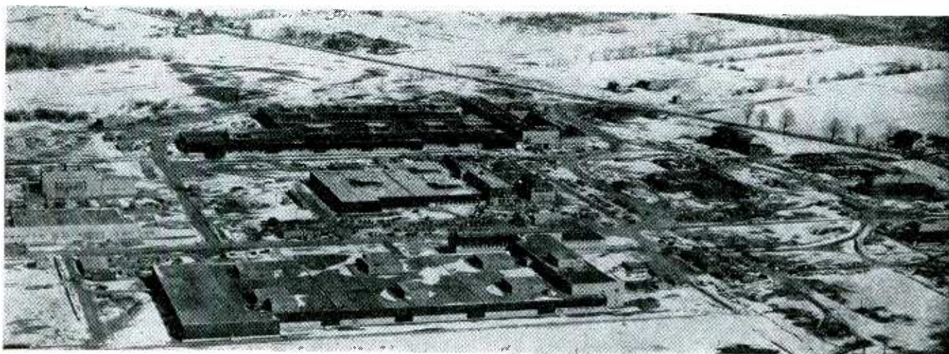
Production of radio transmitters is now under way in the large building in the foreground, first of the nine units of General Electric's mammoth electronic manufacturing and research center to get under way. Construction status early in March is shown in this air view of the 155-acre tract located about 5 miles north of Syracuse, N. Y.
