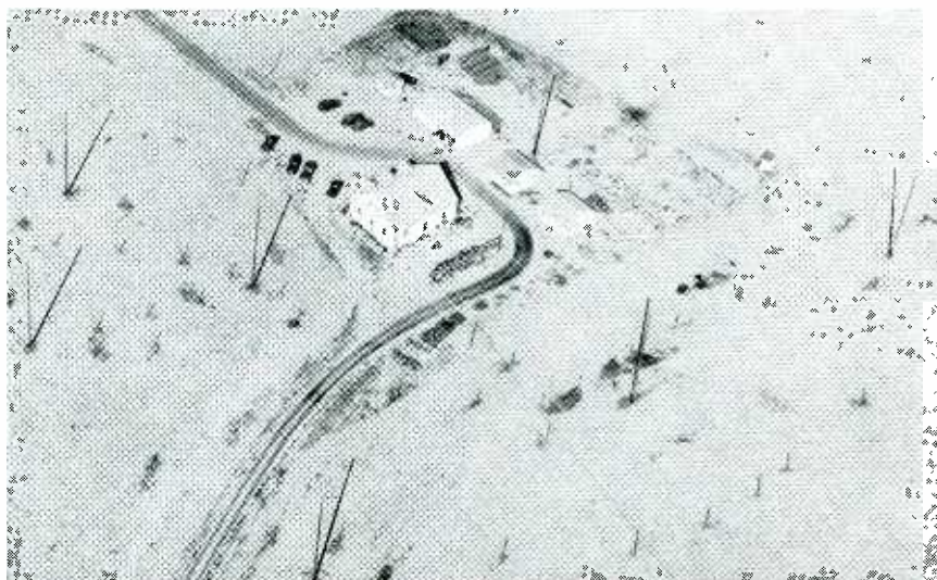
Santa Ana Monitoring Station, showing disposition of a few of the antennas
