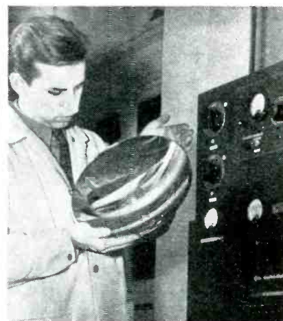
Spherical mirrors for projection television receivers are aluminized by evaporation in vacuum chambers
