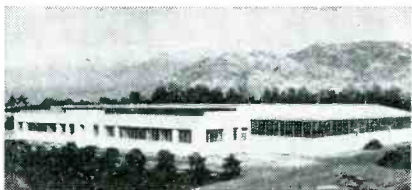
Colonial's new California plant
