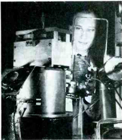
Setup at Battelle electronic laboratories for measuring characteristics of glow discharges at reduced pressures in gases of high purity
