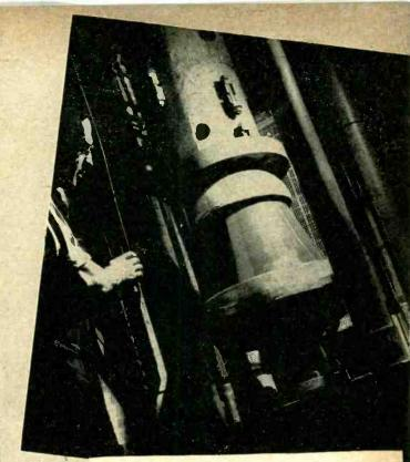
"A million pounds on a teacup." This Lapp compression cone is a supporting insulator for a guyed-mast radiator. With a wall thickness of  $2\frac{1}{2}$  inches of porcelain, it is proof-tested at 1,500,000-lb. loading. The unit withstood 3,000,000 lbs. on design test.
