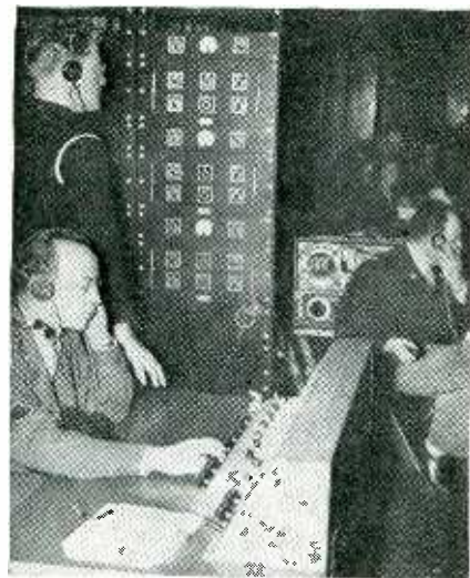
American electronic equipment at the Nuremberg war crimes trials includes an IBM switchboard at center, Western Electric control board in foreground, and a Frederick Hart recorder at right
