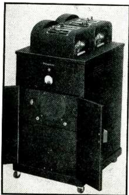
FIG. 1—Dictaphone Belt Electricord recorder-reproducer records for one hour
