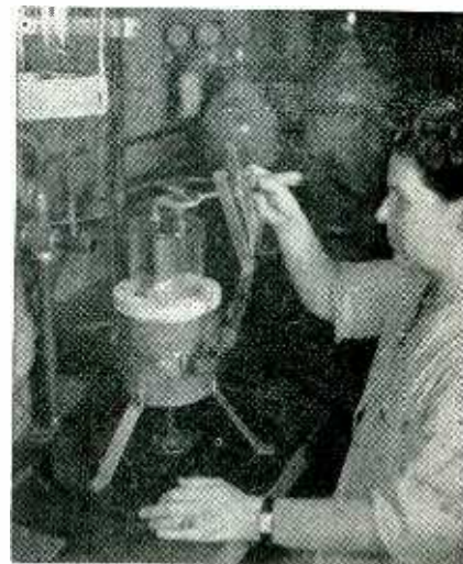
Plate connectors are brazed to the caps on 833A transmitting tubes at the Dobbs Ferry plant of North American Philips. The plastic protective screen shields the operator from flying glass in the event the tube shatters
