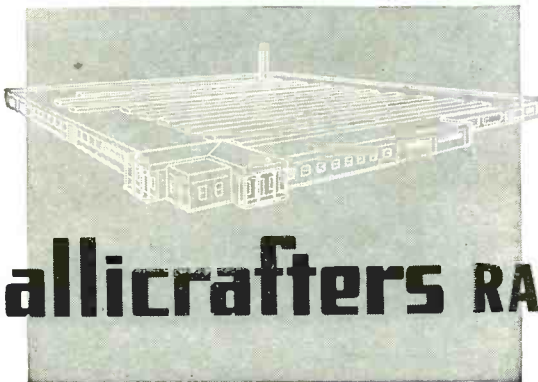
HALLICRAFTERS NEW $600,000 HOME NOW UNDER CONSTRUCTION.
