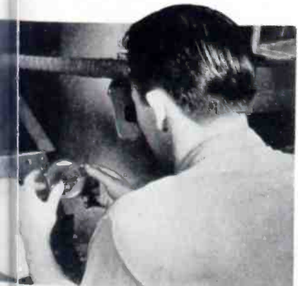
...the entire glass bulb with the help of special light. This device shows up stress on the glass which might be created during shaping operations.
