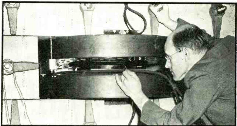
A close-up of the rheotron with W. F. Westendorp of the G-E Research Laboratory making an adjustment
