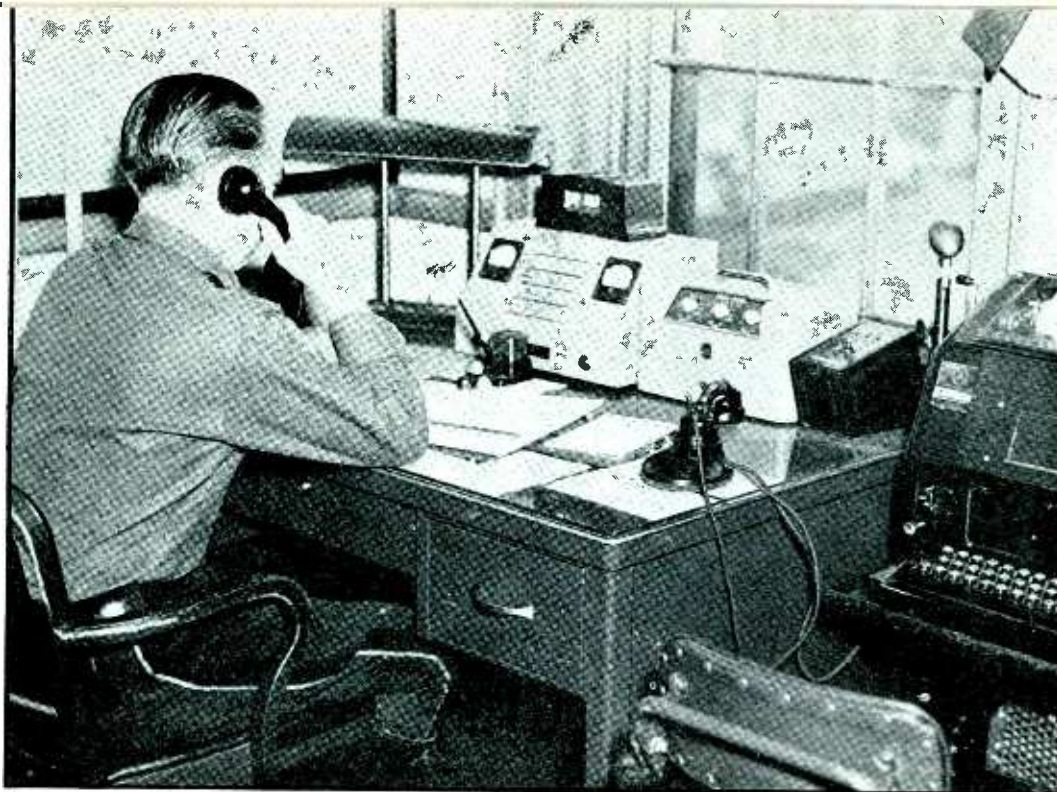
Fig. 10—The control unit at headquarters. The transmitter is put in operation when the operator pushes a button on the handset. Transmission occurs on 39,500 kc, reception on 39,180 kc
