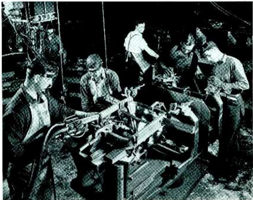
Electronically controlled spot welders in the shape of guns are now widely used to assemble automobile bodies. The operator pulls a trigger which starts a series of accurately timed current pulses. An operator may join 20 parts in 150 places in less than a minute on this jig for a radiator and grille assembly
