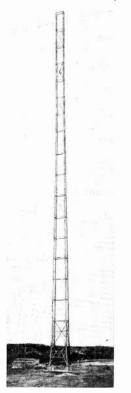
top, and base width is made unusually narrow but with perfect safety because of the low mechanical loads imposed on the insulators.
