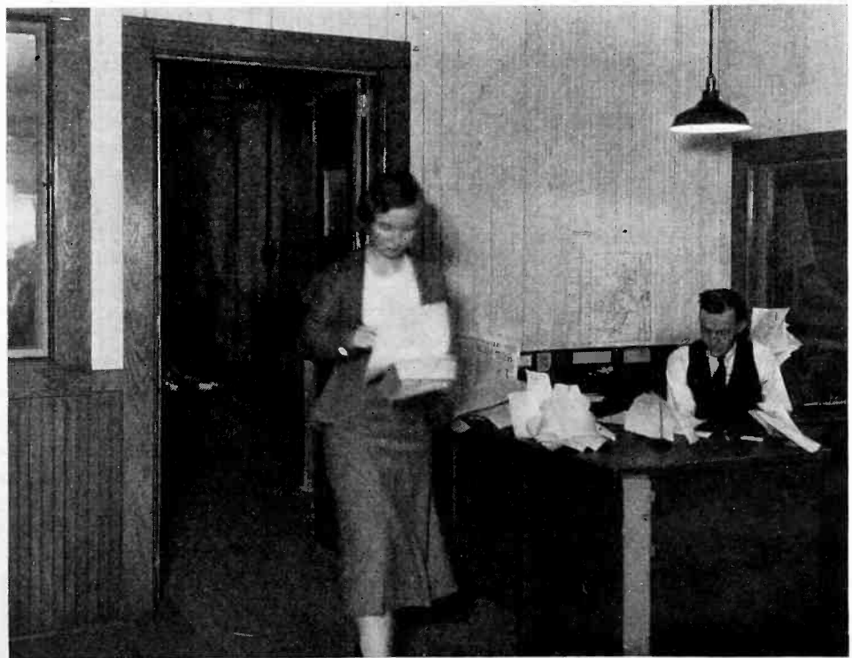
The New Britain (Conn.) Herald has installed this door between its print-shop and editorial offices. Light-beams on both sides control door from both directions. H. H. Raymond, Berlin, Conn., was engineer
