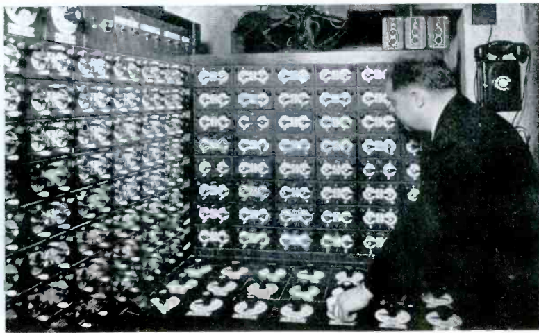
BELOW—The electron-tube control of the stage lighting in the great new Chicago Civic Opera House, using selsyns, and thyatronns.
