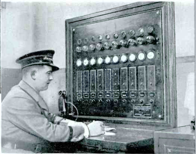
Above—Electric Eye—Traffic Control Room on the Ambassador Bridge at Detroit. System illustrated devised by Benjamin Cooper of New York.
