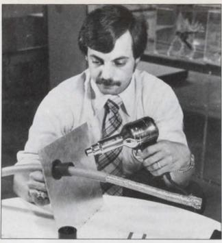
3. The hot-air gun is the most popular heating tool for shrinkable material. It can be used to shrink a feed-through seal around a heavy-duty control cable (left) or
