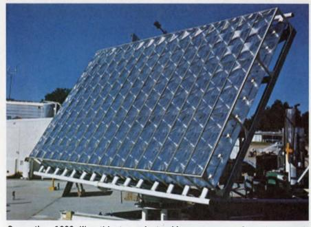
**Generating 1000**  $W_p$ , this two-axis tracking array uses fresnel lenses to concentrate solar energy 60 times. Lenses are 80% efficient; grooves are turned inward to prevent dirt from accumulating.
