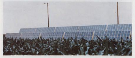
**The largest photovoltaic installation yet** is this 25-kW<sub>p</sub> array at an irrigationwater pumping station in Nebraska.
