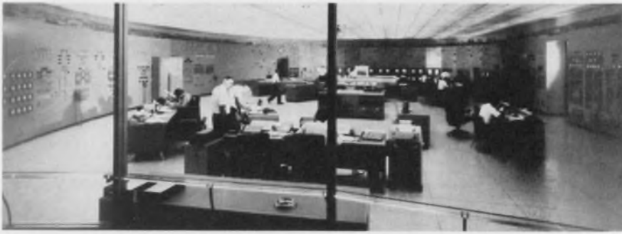
Technicians monitor and control power flow through 325 substations from Con Ed's Energy Control Center.
