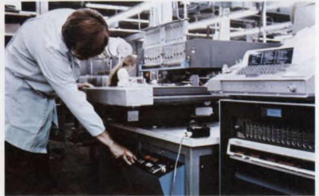
Control of processes and monitoring of quality control are performed in many plants by minicomputers such as this one from Digital Equipment Corp.
