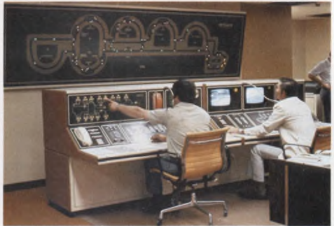
Computer displays tell Airtrans controllers how well every aspect of the airport's ground-transportation system is working so they can interact with it.
