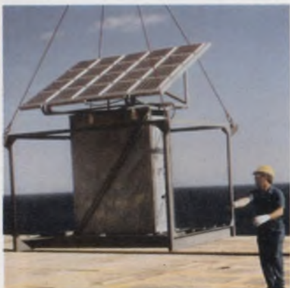
Panels of solar cells, by Solar Power, will provide electricity for horns and lights on this offshore platform.
