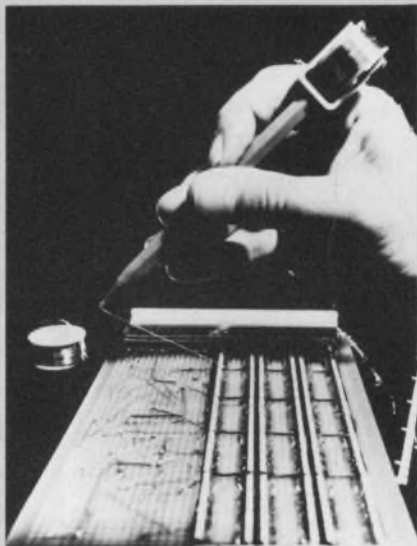
A special pen that issues wire from its tip speeds up circuit construction in Siemen's new breadboard system.
