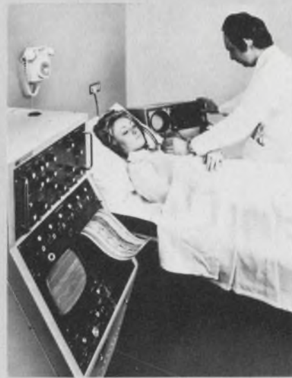
Echo interference module is used with a fiber-optic medical recorder to measure heart valve movements.
