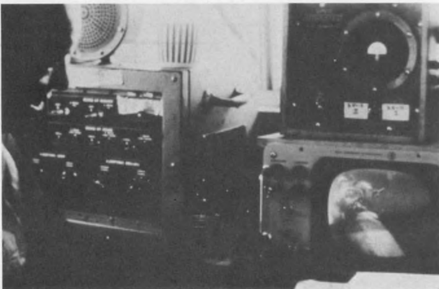
Westinghouse surface station has an underwater TV monitor, telephone switchboard and a terminal for each diver's oxygen sensor telemeter.
