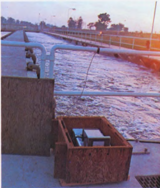
Brady brought his Beckman dissolved-oxygen meter right to his aeration tank, dropped its sensor into the effluent, and plugged it in. The instrument worked so well, it turned up a testing flaw: bacteria used the oxygen.
