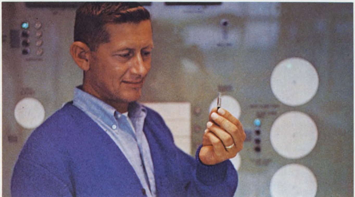
John Brady mourns the loss of yet another banana bulb. The bulbs apparently get overheated inside their colored buttons. Brady long ago gave up replacing banana bulbs, and the panel behind him, installed by Honeywell, is now
