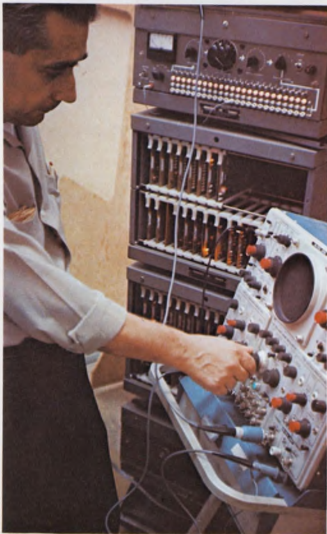
In case of failure, neon lights tell a rapid-transit repairman which printed-circuit card malfunctioned. Here, a technician checks the repaired card in a "working" simulation. A foam-gasketed lucite plate covers the front.
