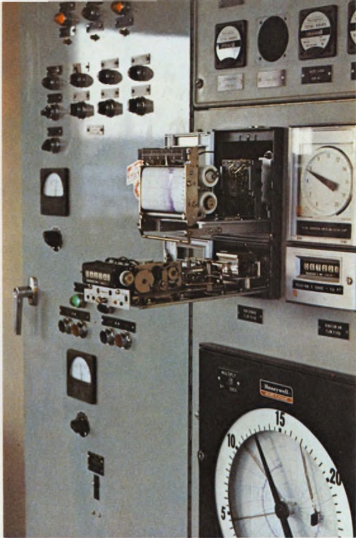
This strip-chart recorder is supposed to measure sewage flow. Its rollers, however, fail to pull paper past the pen. Below it, an electronic integrator records total sewage. Unfortunately, it loses about a million gallons a day out of about six million that the plant processes.
