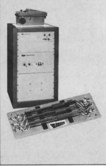
Acton Laboratories' latest Rayspan<sup>TM</sup> spectrum analyzer designs combine sharp, stable, magnetostrictive filters with solid state switching to make real-time analysis practical in rugged environments. A frequency-amplitude display allows for operator analysis or digitization of the output for computer analysis. Great flexibility is possible in filter bandwith and analysis band. Current Rayspan designs cover 1 Hz to 100 Hz in filter bandwidth, and 30 Hz to 50 KHz in analysis band.
