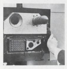
5. Car coupler contains large electrical connector. Dixie Howell presses plate to remove shield.
