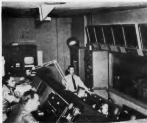
Control room of the Air University's closed-circuit television system, where questions from students are relayed to the TV lecturer while he is on the air.
