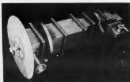
S-Band monopulse tracking feed, integral L-band monitoring dipole
