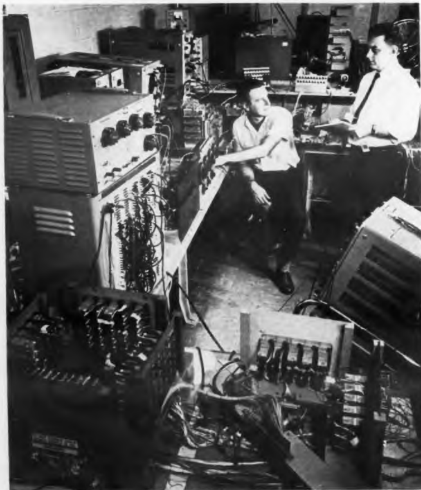
Fig. 1. Breadboard for present Mark I version of Bendix airborne digital computer is being built up with "first-generation" production modules being used as "plug-in logic." Some of these modules can be seen in the foreground. The unit in the left foreground is the computer's arithmetic unit. The input-output unit is along the bench to the left and the fast memory units are on the bench at the rear. Engineer Rod Simister is standing.
