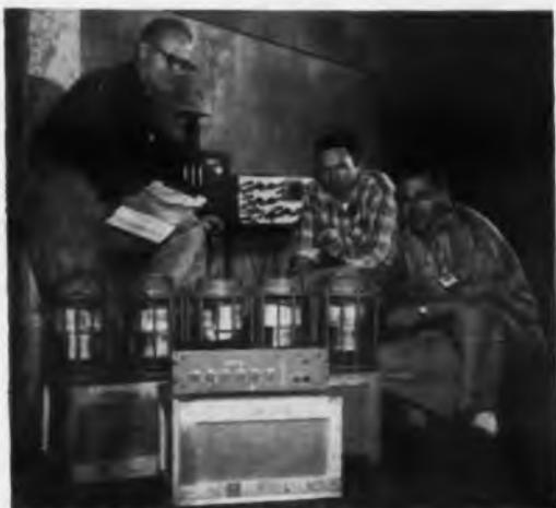
Underwater current speed transducers and some of the surface equipment is displayed by Roy Gaul, of Texas A & M, left, Henry Walker, vice president of Hytech Corp. and Don Crezler, president of Hytech, right. Current devices are Savonius rotors, standard velocity measuring device.
