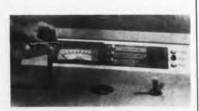
**Transistorized digital circuitry** counts output of scintillation counter which gives indication of radioactivity in patient's blood sample. Accurate measurements are first made of background radiation in patient's blood before he receives injection of measured dose of radioactive iodine.
