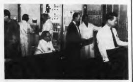
Engineers test a new system that will check out the launching of this country's first Saturn booster later this year from Cape Canaveral, Fla. Monitoring more than 100 functions, the system will automatically stop the launch sequence in the event of any malfunction. It was developed by the Guidance and Control Div. of the National Aeronautics and Space Administration.
