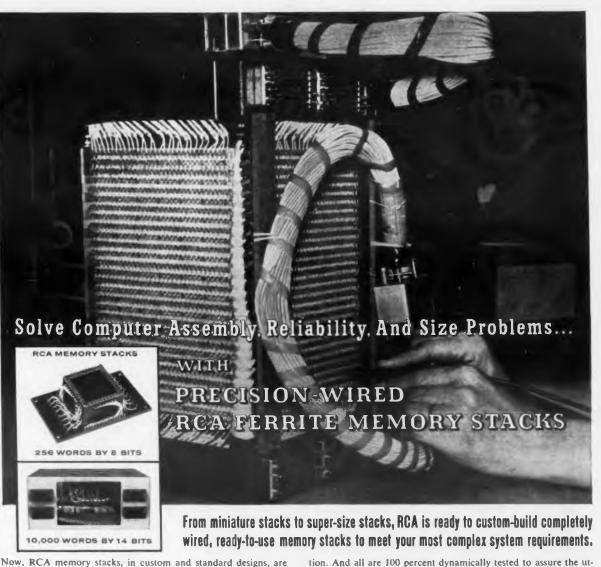
available to help you solve computer assembly problems and meet today's exacting performance specifications. Incorporating RCA ferrite memory cores and planes, with specified wide margins of operation...up to 8 percent, ...RCA stacks can cope with broad variations in power levels.
