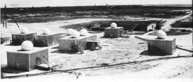
attery of precision radar antennas—part of the Mark II system—permit the Air Force to track missiles with incredible cy. The system tracks a missile by transmitting radio signals to a small airborne transponder which beams a continuous back to earth. This signal is captured by these parabolic receiving antennas and sped into a computing system which ttes the missile's flight progress on a large plotting board. Agusa Mark II was designed and built by Convair/Astronautics.
