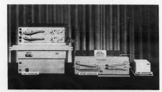
Three generations of guidance computers designed by Arma illustrate the progressive size reduction achieved. The first generation computer is the present Atlas ICBM inertial guidance computer. The second generation computer, not yet assigned to a specific project, uses circuitry embedded in foamed polyurethane. It was developed under Air Force contract. The third generation computer is the microminiature unit now in development.
