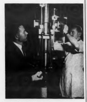
Experimental model of 24-megawatt superpower klystrons, being developed by Sperry Gyroscope Co., Great Neck, N.Y., for a proposed two-mile-long atom smasher, is assembled by Sperry engineers. Energies of up to 10 to 20 billion electron volts are expected to be achieved by driving relatively lightweight electrons along a straight path. Six tubes will be delivered to Stanford University later this year. The accelerator of the atom smasher will require 240 of these klystrons.
