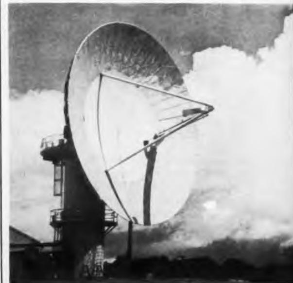
Maser amplifiers operating at X band track reentry vehicles at 200-mile range from this Lincoln Laboratory
