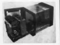
This industrial potentiometer, known as the Electronik 17, incorporates an electromechanical strain gage as the rebalancing element. Infinite resolution is obtained by elimination of the conventional slide-wire. All critical components are isolated within an electrical shield. The unit has one true reference junction compensation for all types of thermocouple actuation. Transistorized plug-in control units are available up to a maximum of eight set points for zone control.
