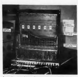
Learning machine of perceptron-type built at Aeronutronic solved problems in Boolean logic equivalent to pattern recognition problems. Machine was test vehicle for biax-type magnetic integrators wanted by Navy for perceptron program at Cornell Aeronautical Laboratory. Larger version of learner under construction at Aeronutronic will also use magnetic integrators. If performance is satisfactory, still larger version, capable of useful work, will probably be built.
