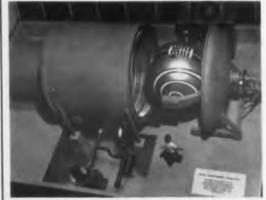
**Space environment simulator** (CVPR-2997), as depicted in scale model, will test payloads nearly 8 ft in diam by spinning and rotating them to duplicate their positions relative to the sun.
