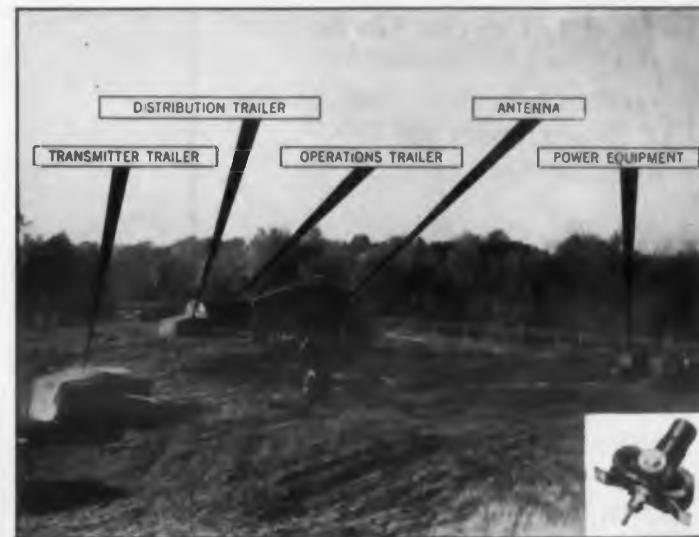
AN/FPS-8 high-power search system by General Electric, used primarily in aircraft control and early-warning operation. The complete mobile version (AN/MPS-11A) shown here, can be airlifted or carried on nine trucks and two trailers.
