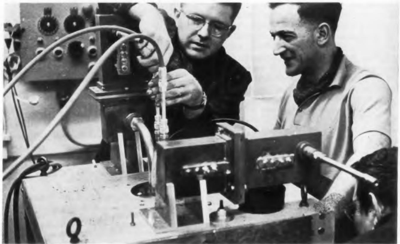
**Project Echo** receiver uses this maser, giving low noise reception considered virtually impossible to achieve a short five years ago. Other breakthroughs like this should permit much more efficient bandwidth utilization than can presently be foreseen.
