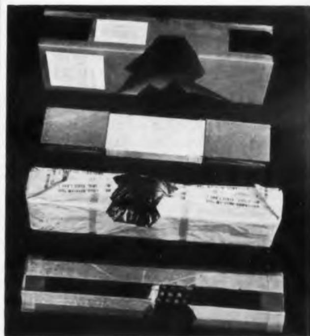
Packaging of component boards with parts soldered in place for shipment is illustrated. This interior package is wrapped in six sides with rubberized hair and packed in a larger exterior container.
