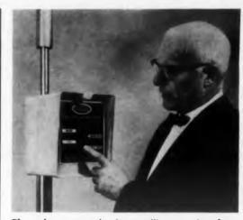
The solar-powered safety satellite transmitter for a highway emergency calling system is demonstrated by H. Leslie Hoffman, president of Hoffman Electronics Corp. By pressing any of four buttons-for police. ambulance, fire truck or service truck—a motorist can transmit a coded radio message summoning help.
