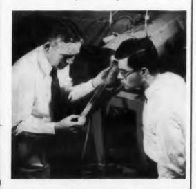
Scientists at Bell Telephone Laboratories, New York, inspect an ingot of gallium phosphide. Bell is developing methods of growing single crystals of a transparent semiconductor, gallium phosphide, and studying its properties. These studies will help in the basic understanding of high-energy-gap semiconductors. The material is transparent, making it possible to observe visually the differences which take place under varying conditions of doping and electron density.
