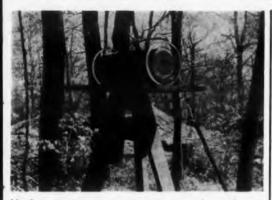
Nuclear precession magnetometer takes a dry run in the woods behind the Lamont Geological Observatory. Device consists of a water-filled cylinder surrounded by energizing and sensing coils.
