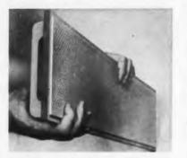
Melamine Laminates. Glass cloth or cotton fabric impregnated with melamine formaldehyde resin. Taylor melamine laminates have superior mechanical strength and are especially desirable for their arc-resistant qualities. Good flame and heat resistance, good resistance to the corrosive effects of alkalis and most other common solvents, besides other favorable characteristics. Typical applications include arc barriers, switchboard panels, and circuit-breaker parts in electrical installations.
